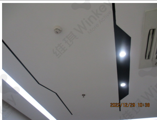
Fire sprinkle and smoke detector.JPG
